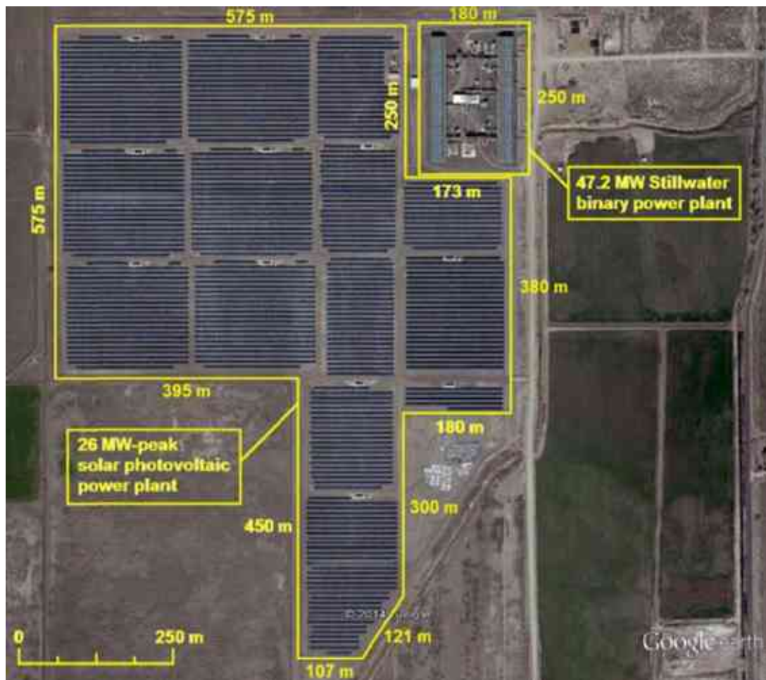
Figure 13-1: Aerial view of Stillwater combined power plant ( DiPippo, 2016c )
